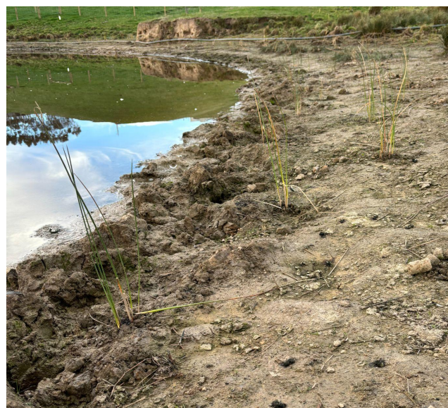
Topsoil spread on dam wall edge to help plant establishment
